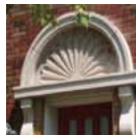
Doorway Arch Corbels
